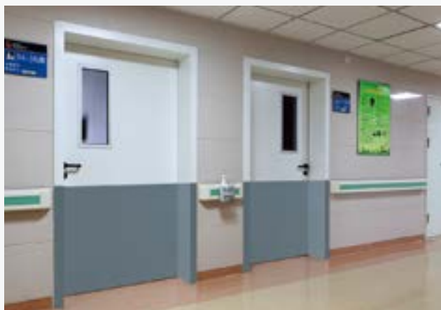
Protection plate is not only decorative but also antibacterial and fire-proof.
